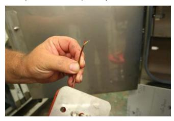
5. Splice the new thermocouple wires together with the old thermocouple wires coming from the smoker connecting the red wire to the red wire and the yellow wire to the yellow wire. Use nylon insulated wire splices (butt splices) #22 - #18 AWG (221°F minimum temp. rating, 600 V max). CAUTION: The correct splice is critical for good wire connections that are necessary for a proper signal path back to the thermostat.
